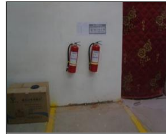
Photo of the inside of the main production hall Fire extinguishers 4.JPG
