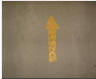
Photo of the inside of the main production hall Evacuation arrow.JPG
